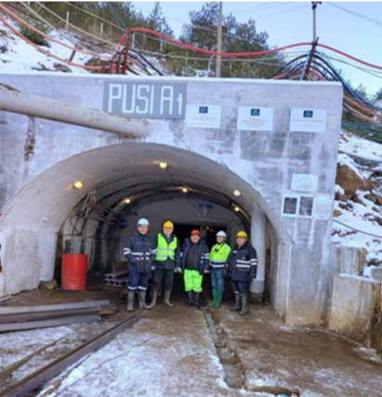
Fig No.6 Shaft A1 Entrance Bulqiza North
