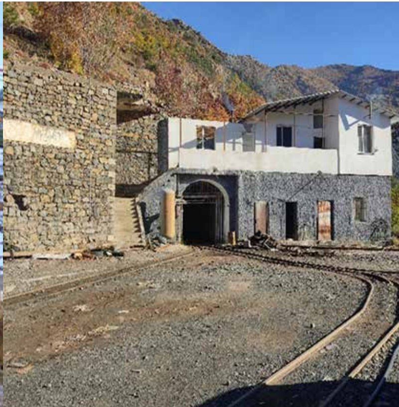
Fig No.7 Main Level 41 Entrance Bulqiza North
