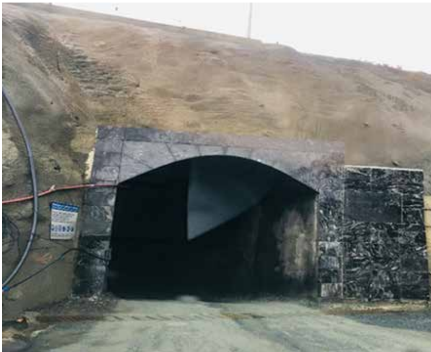
Fig No.12 Fig Main Ramp entrance Munella Mine
