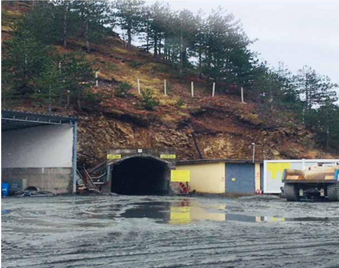
Fig No.11 Main Ramp entrance Spaç Mine
